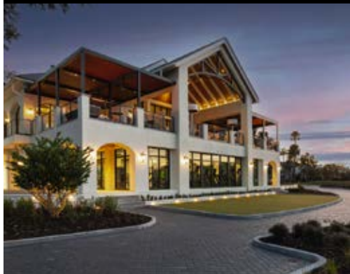
Brasfield & Gorrie, LLC The Plantation - Clubhouse Renovation Ponte Vedra Beach, FL
