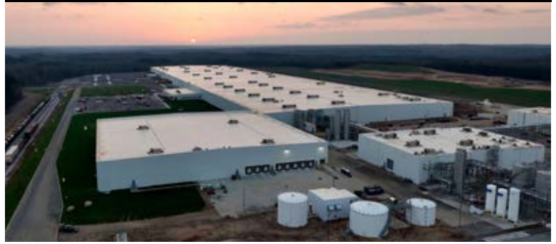
Project Eco Fort Lawn, SC
