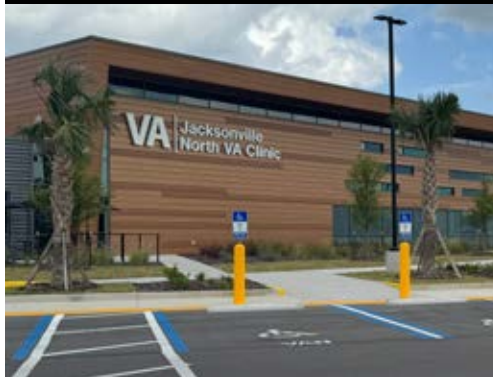
Campbell Plumbing & Mechanical Contractors Southeast, Inc. VA Outpatient Clinic & Domiciliary Jacksonville, FL
