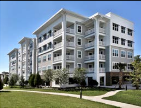
Danis Vicar's Landing at Oak Bridge Flats III Ponte Vedra, FL
