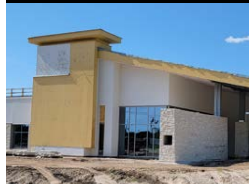
Allstate Steel Company Baptist Nassau Crossing MOB & FSED Yulee, FL
