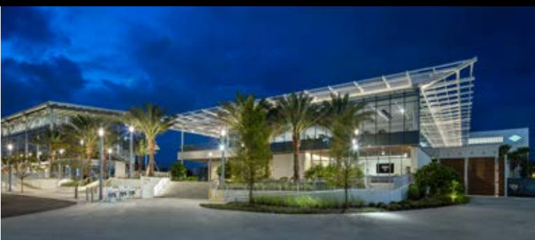
Jacksonville Jaguars Sports Performance Center (Miller Electric Center) Jacksonville, Florida
