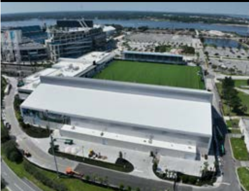
Register Roofing & Sheet Metal, Inc. Jacksonville Jaguars Sports Performance Center Jacksonville, FL
