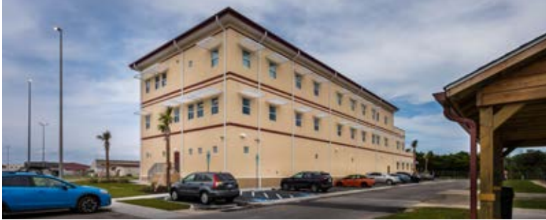
Fort Macon Hurricane Rebuild Atlantic Beach, NC
