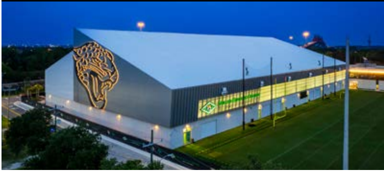
Miller Electric Center Jacksonville, FL
