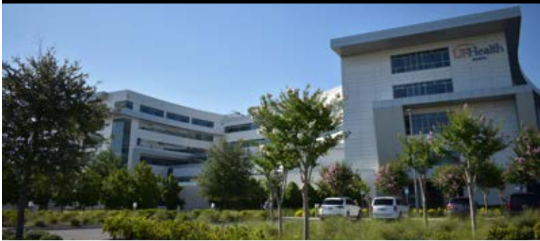
UF Health North Tower Phase 3 Allstate Steel Company Jacksonville, Florida
