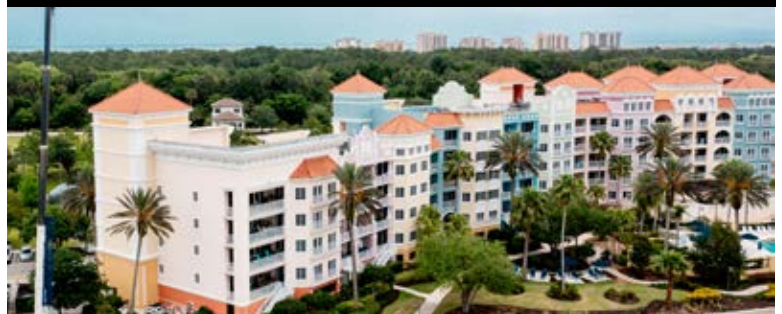
Yacht Harbor Condominium Roof Replacement Palm Coast, FL
