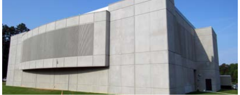
Joint Special Operations Command - Special Operations Facility Fort Liberty, NC
